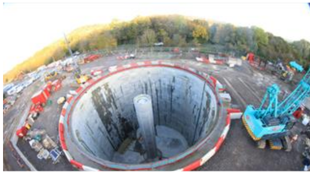
Storage tank installation at Stroud
