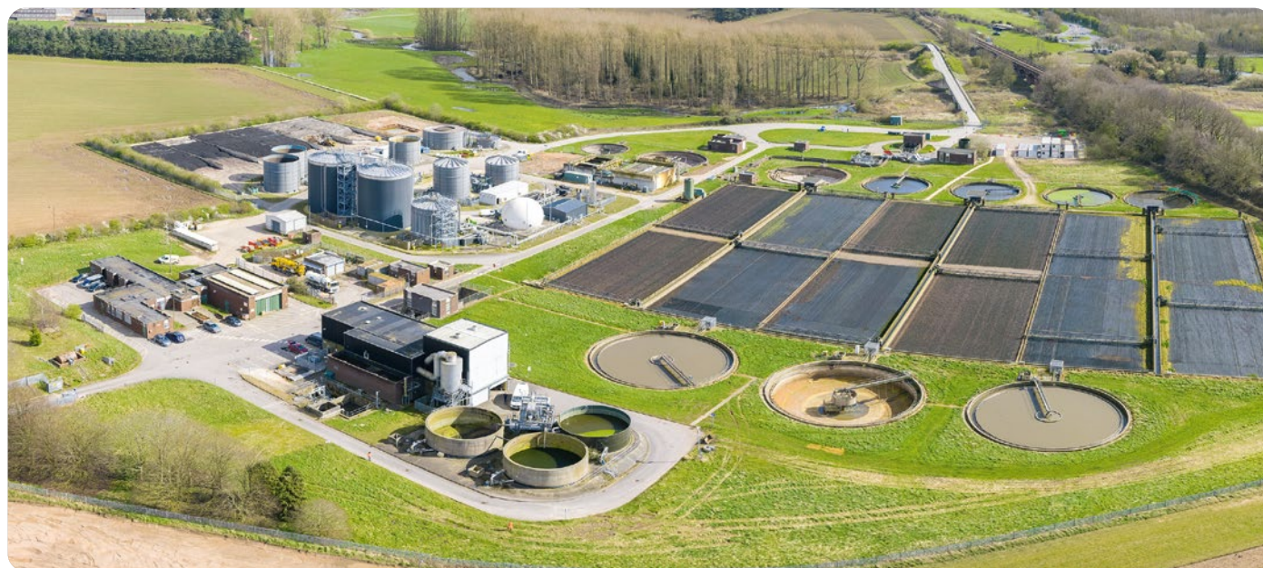
Worksop wastewater treatment works
