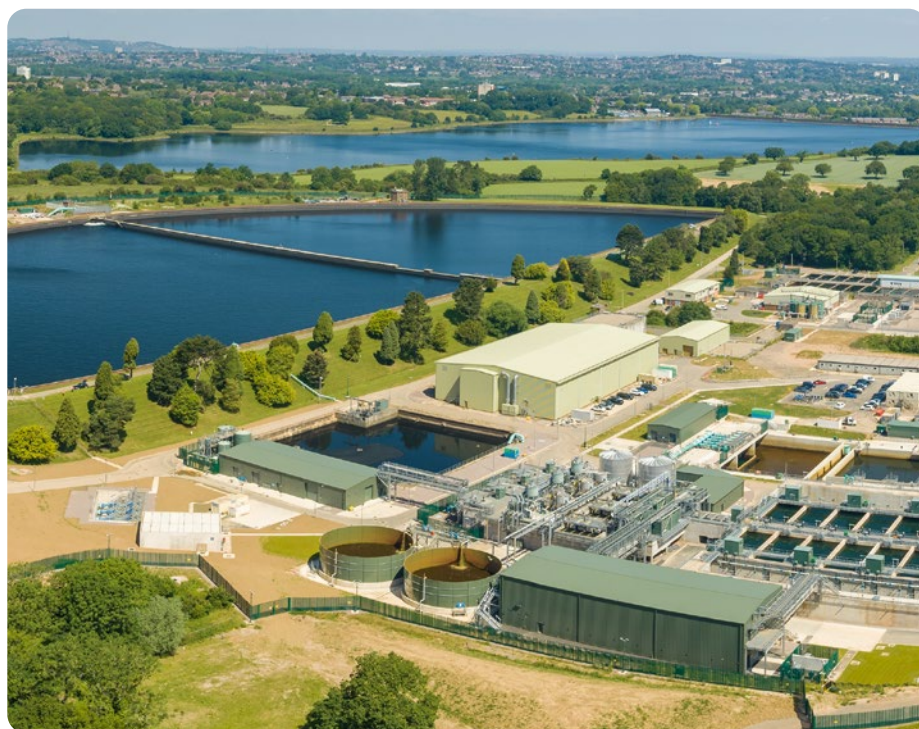
Frankley water treatment works
